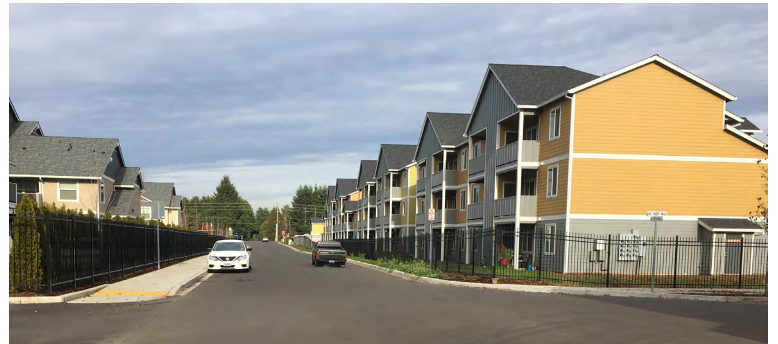
A street that has a sidewalk on only one side is less pedestrian-friendly and accessible than sidewalks on both sides.
